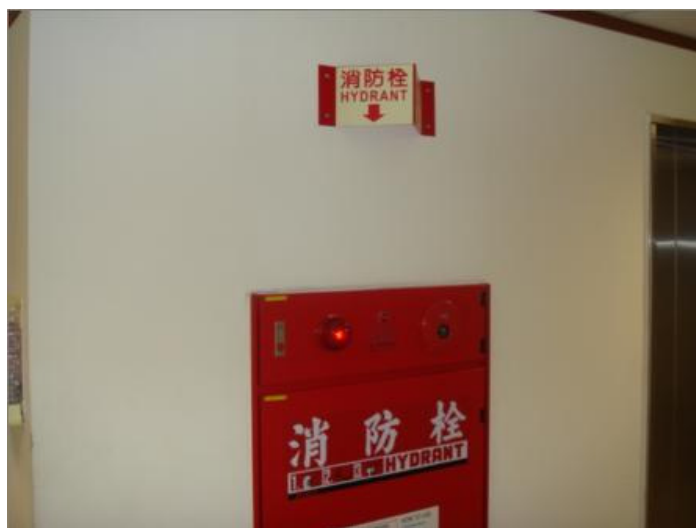
Fire Hydrant and Box added with 3D marking
