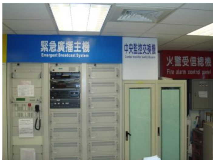
Established the Monitoring Center
